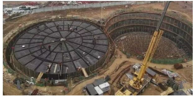
Fig. 10 Model of underground granary silo with backfilling 2:8 lime soil (Wang et al., 2022)
