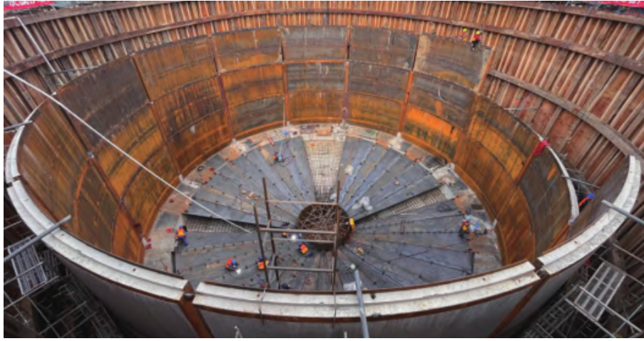
Fig. 8 On-site construction of prefabricated underground granary (Zhang et al., 2021, 2024)
